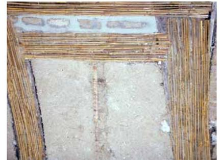
*Reed matting St70 on wooden beams of a half-timbered wall*
