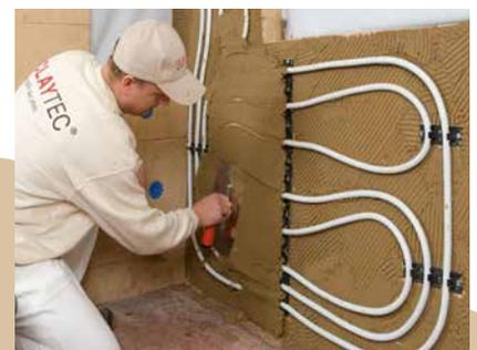
*The undercoat plaster is smoothed over the pipe clamp*
